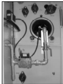
Figure 5.3: IS Series Gas Heat Detail
